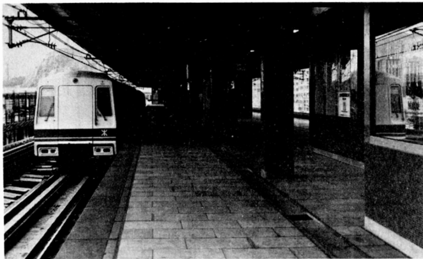
Fig. 5. Kowloon Bay station: platform and canopy
