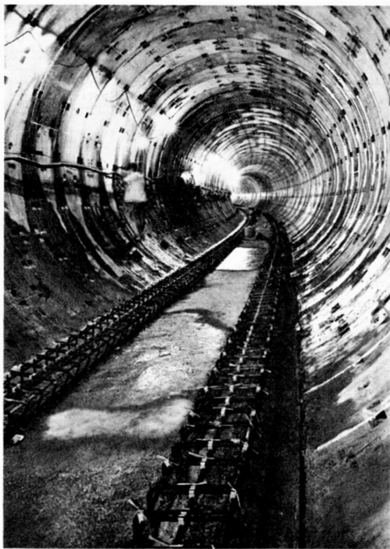
Fig. 23. Rail plinth starter bars
