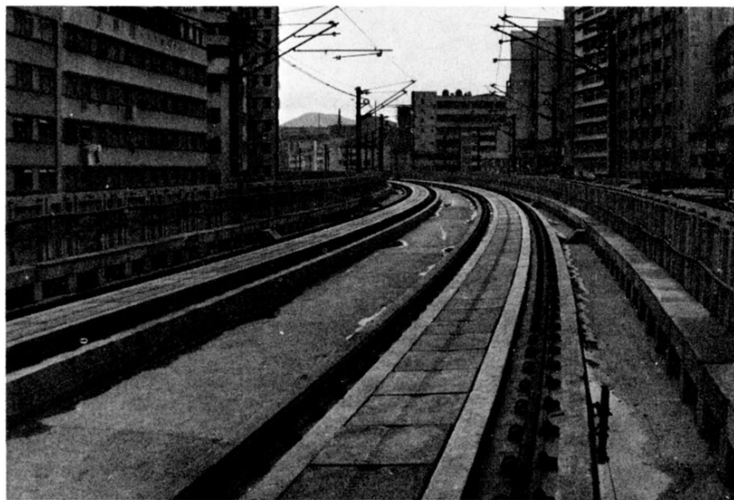
Fig. 22. Track with derailment upstands
