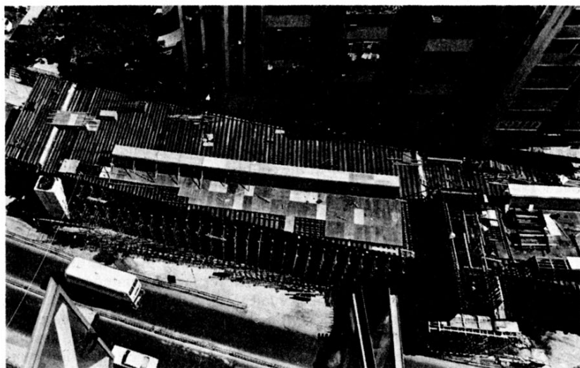
Fig. 4. Falsework on section F
