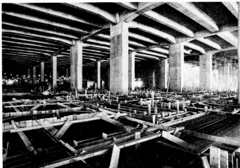
Fig. 13. Kowloon Bay Depot: floor construction
