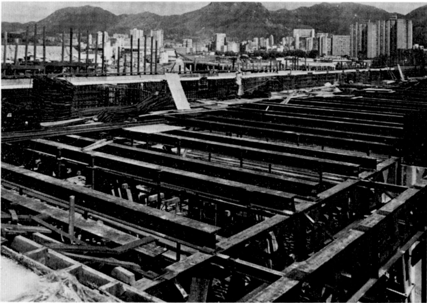
Fig. 18. Kowloon Bay Depot: falsework for podium roof
