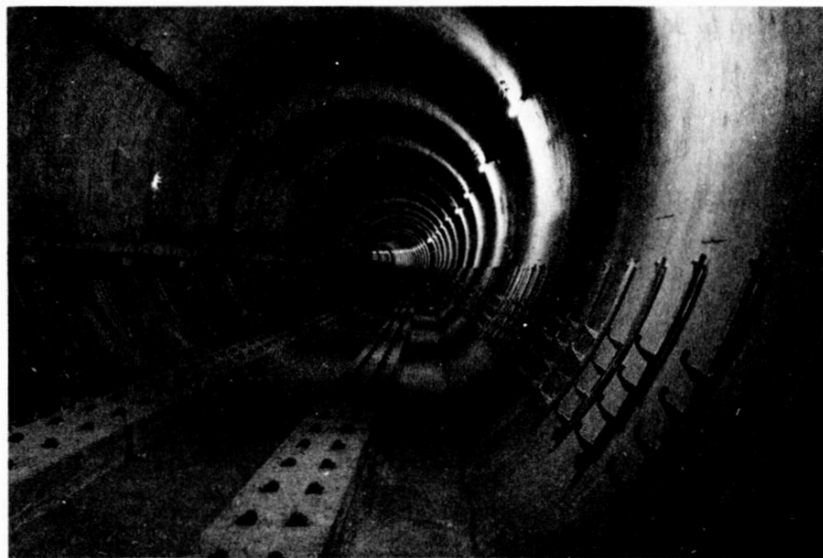
Fig. 29. Track plinth completed
